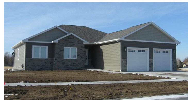
(top and bottom) Geneva before and after construction.
