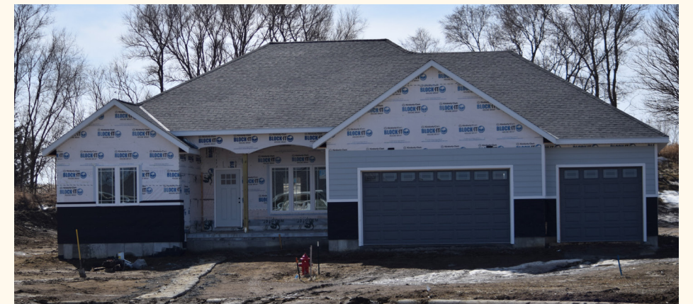
Single-family homes in Wakefield constructed with support from the RWHF.
