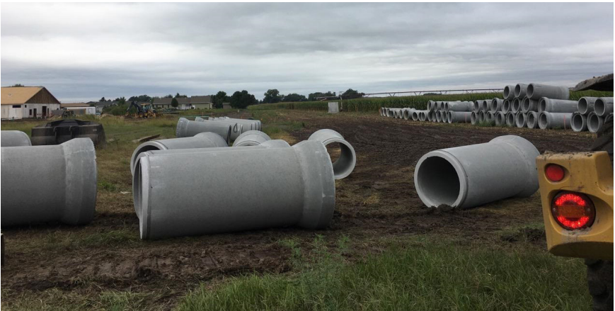
Piping for Burwell’s new storm sewers.
