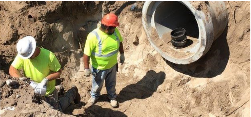
Replacement of the original system with new piping.
