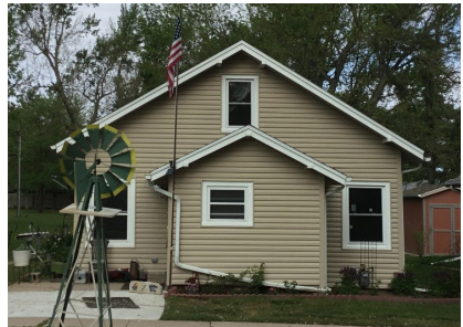
Completed owner-occupied rehabilitation.
