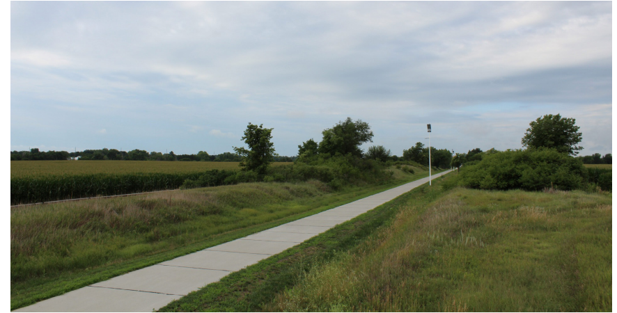
Ongoing development of Pioneer Spirit Trail is expanding pedestrian, bicycle, and exercise routes and encouraging active modes of travel.
