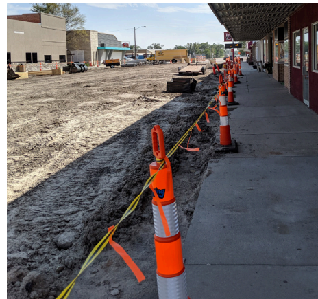
Work underway in Cambridge.
