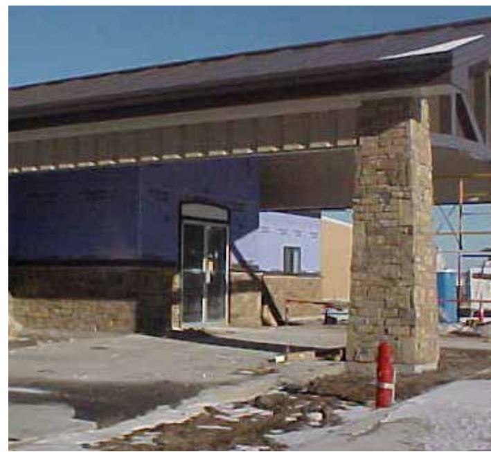
Pilger Community Center under construction.
