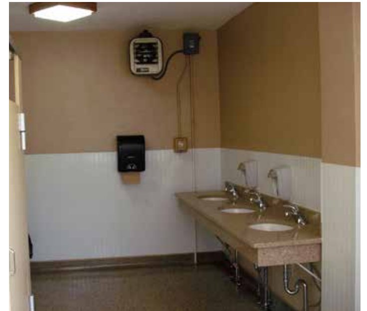
David city restrooms under construction.
