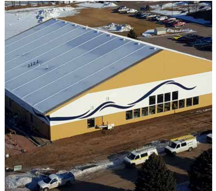
Chadron Aquatic Building under construction.
