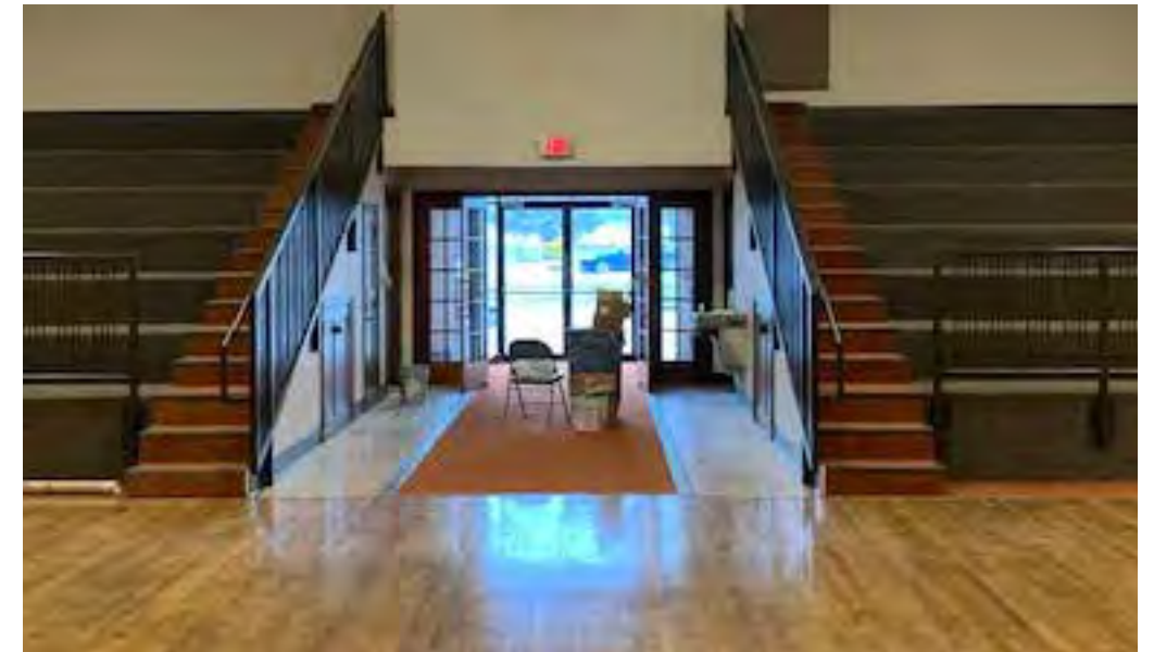
Tekamah Auditorium under renovation.
