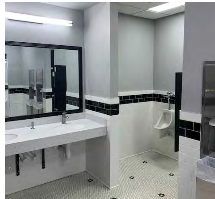
New restrooms in the renovated Tekamah Auditorium.
