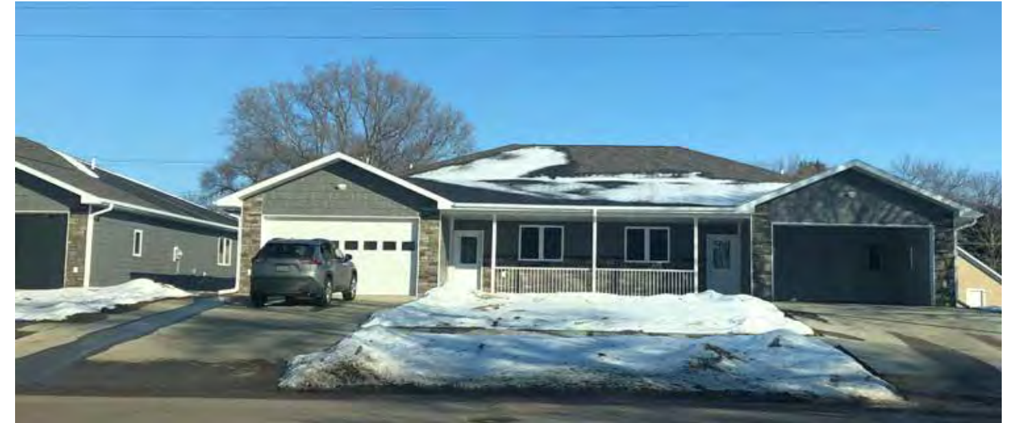
Newly-built rental units in Bloomfield.
