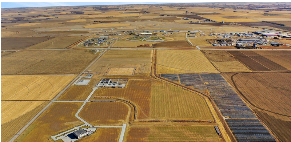
Kearney's Tech oNE Crossing was made possible in part by a $100,000 investment from the Site and Building Development Fund. In 2019, Compute North, a Minnesota-based tech firm with operations in South Dakota and Texas, entered into a $7.65 million agreement to locate at Tech oNE and create 10 new full-time technology and security jobs.
