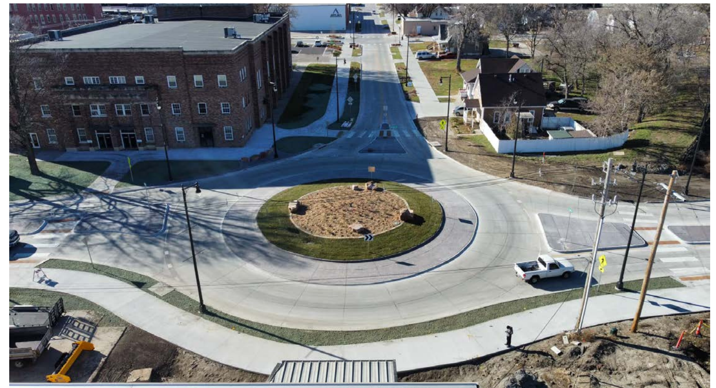
Improvements to Johnson Park in Norfolk. Norfolk received a CCCFF planning and construction award for the project in 2019 and 2020, respectively.
