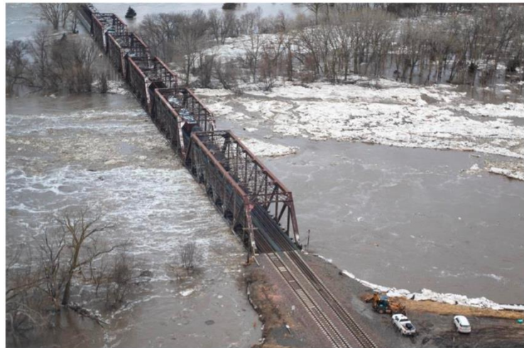
Figure 2-9: Flooded Railway Bridge
