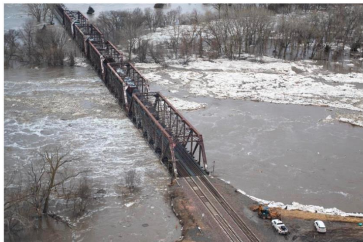
Figure 2-9: Flooded Railway Bridge
