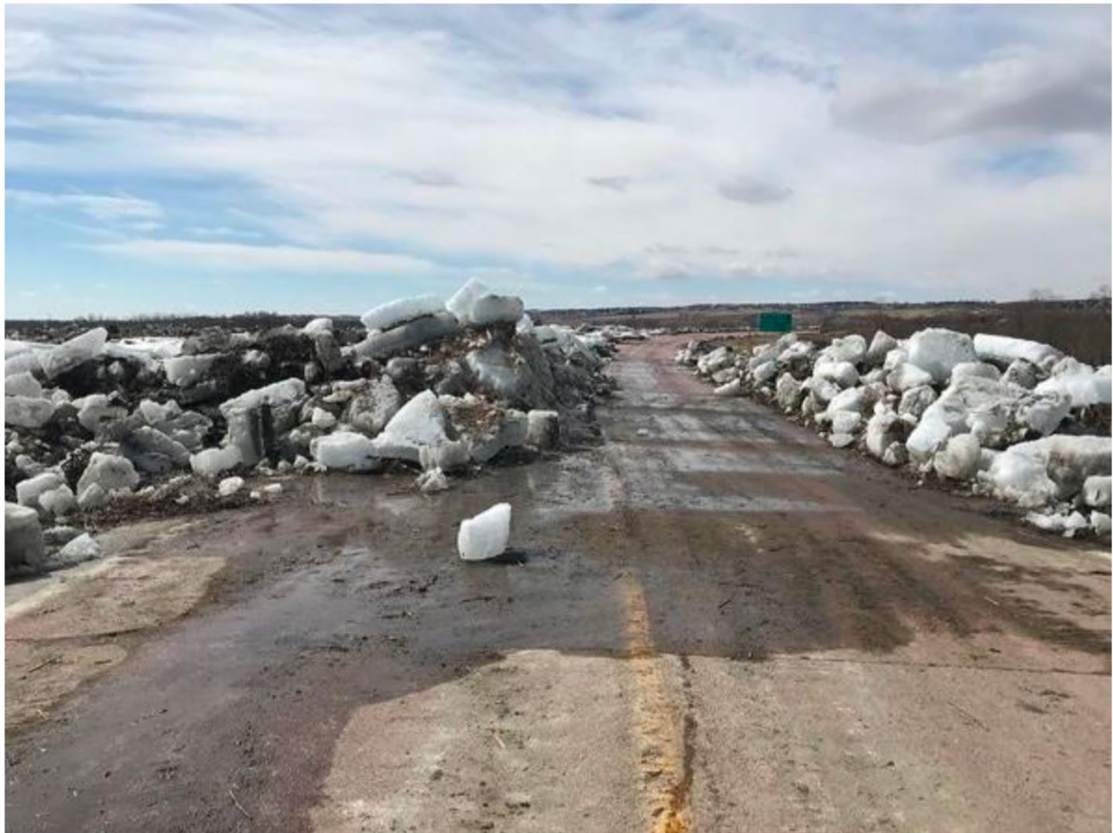
Figure 1-6: Photo of Ice Accumulation after 2019 Disaster
