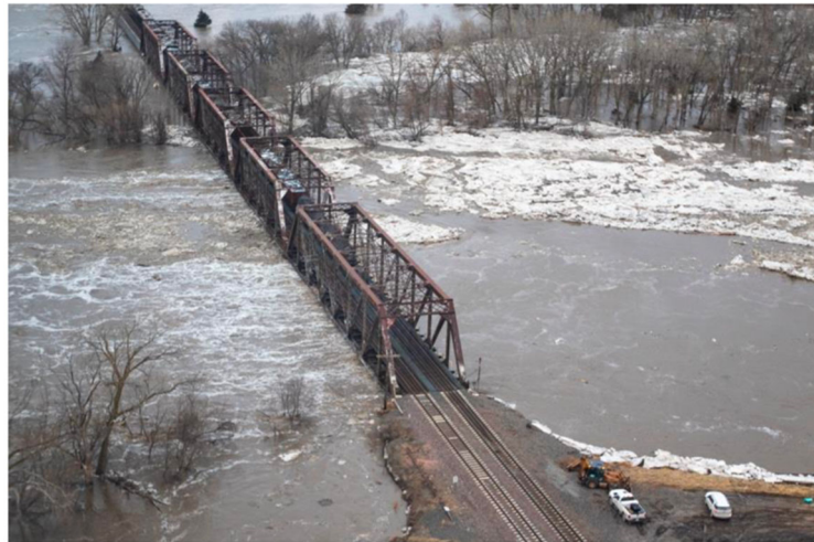
Figure 2-9: Flooded Railway Bridge
