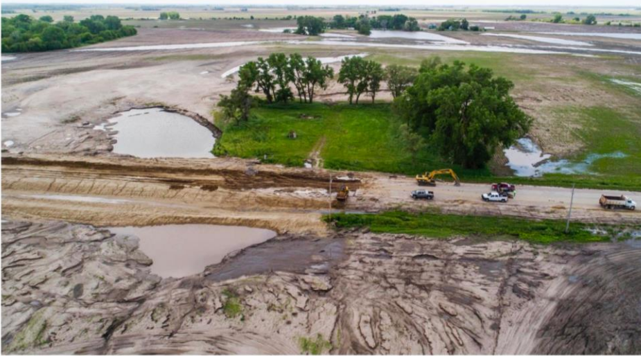
Figure 2-12: Washed-Out Road Under Repair
