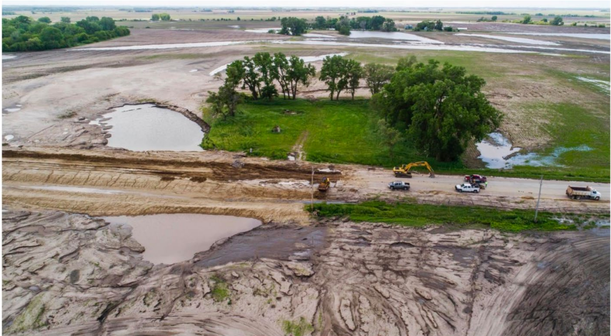
Figure 2-12: Washed-Out Road Under Repair
